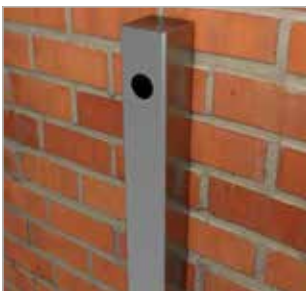
1 Drill a 25mm diameter hole through front wall of post
