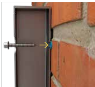
2 Drill rear wall of post with required diameter for fixing and then fix post to wall. Insert appropriate fixing into the wall for affixing post
